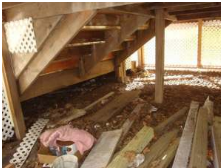
8. FRONT PORCH STAIR FRAMING
